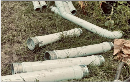
TurboFloc in-pipe treatment before discharge.
